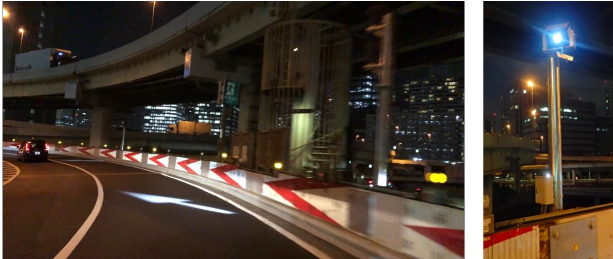
Fig.8 Dynamic lane assignment: a variable indication of lane role by flood light at Tokyo Metropolitan Expressway.
