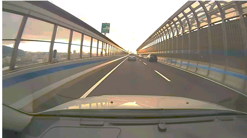
Fig. 9 Level lines and a signboard (Route 3, Hanshin expressway)
